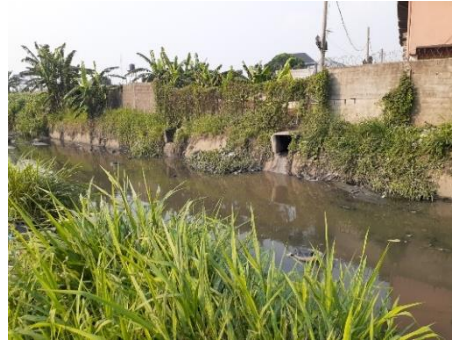
Plate 2: (Location 2): Machanic village by car wash D-line
