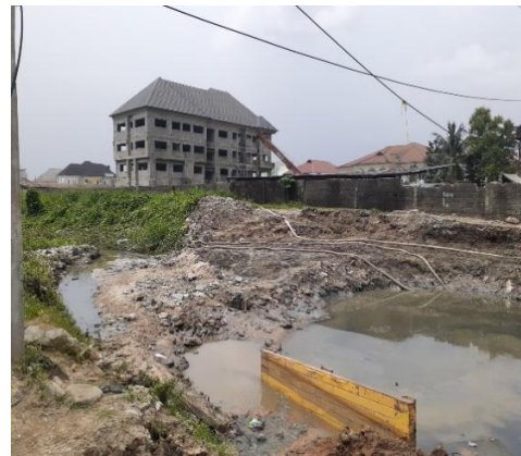
Plate4: (location 4): Tombia Street extension GRA Phase 3
